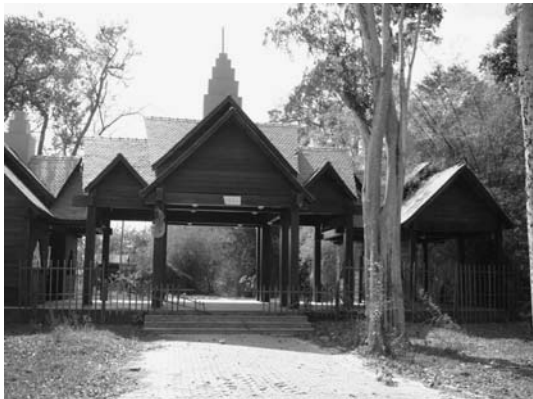
Photo 6 Suspended Spa resort construction
