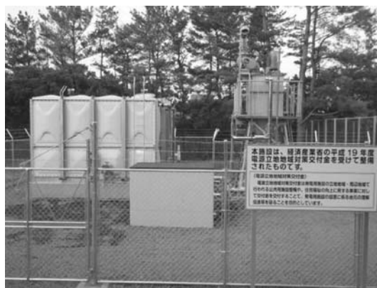
Fig. 3 Facilities of Kamisu-Wakamatsu hot spring source. 図 3 かみす若松源泉の温泉設備
